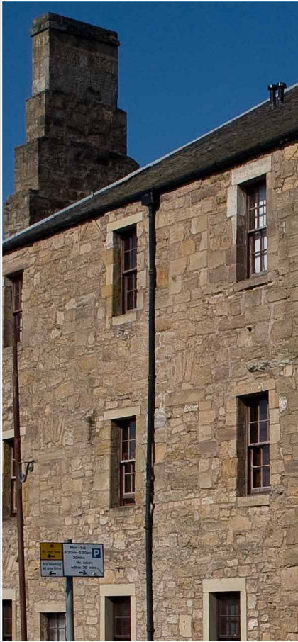
The exposed wall of this 17th-century house in Cupar, Fife, reveals archaeological evidence of a number of blocked openings. The previous mixture of window sizes and levels has been regularised in the current arrangement. © N. Haynes.
