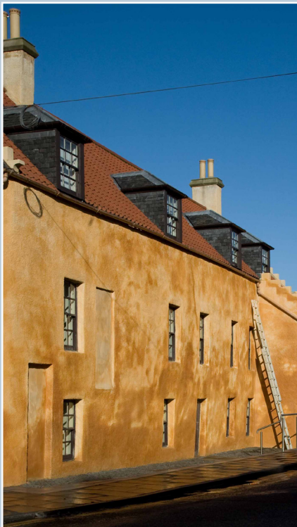
Dymock's Buildings (late 17th century), Bo'ness, were restored by the National Trust for Scotland in 2004. A cement render was removed, the archaeology of the wall recorded, and then a lime harl and limewash were applied. Evidence of former openings remains visible. © N. Haynes.
